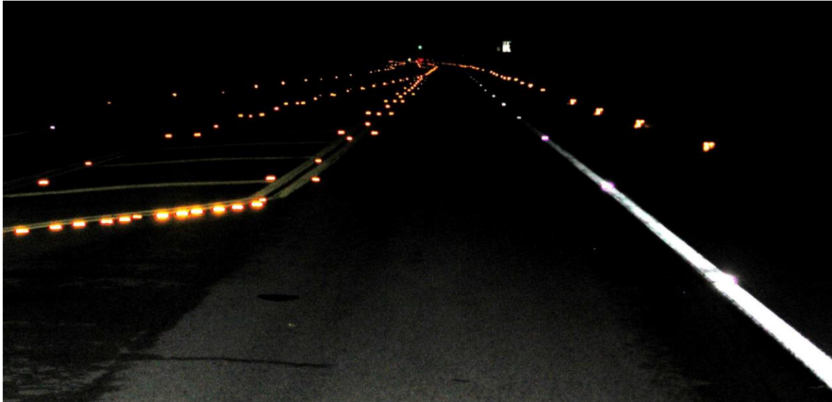
Figure 27. Embedded roadway lighting. These LED lights installed in the pavement are not visible to sea turtles nesting on the adjacent beach and are well received by motorists and pedestrians (Bertolotti and Salmon 2005). Photograph courtesy of Michael Salmon.
